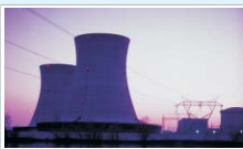
Thermal power station
