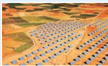
Solar power station
