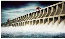
Hydraulic power station
